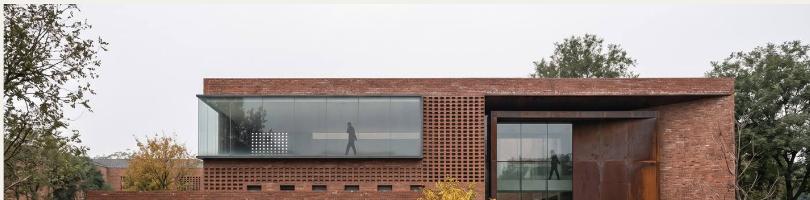
06 Main facade — brick mass, a cantilevered glass room and a weathering-steel entry
