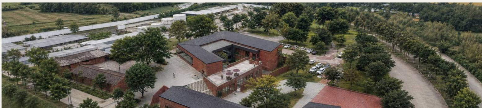
01 The retained brick halls set within fields and tree lines
